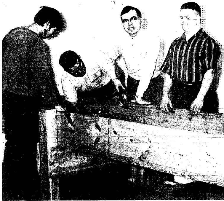
(Above) One of the more extensive projects finished by Center clients was the construction of a feed-bunk. Workshop Director Arthur Magel says the clients are justifiably proud of their good work.
